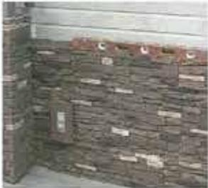
5. Check if the panels are horizontal with a level during installation.
