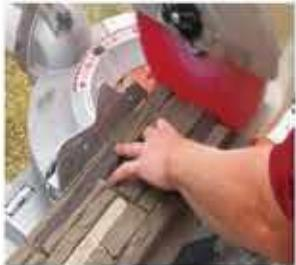
7. Cut the panel with a saw if necessary.
