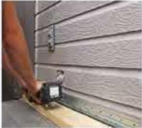
2. Put the starter strip on the bottom of the wall.
