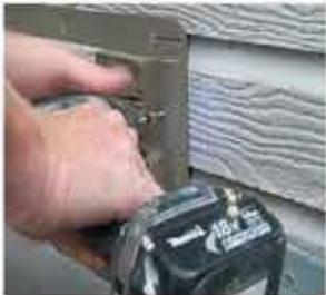
8. Drill the screw through the center of the joints to the wall
